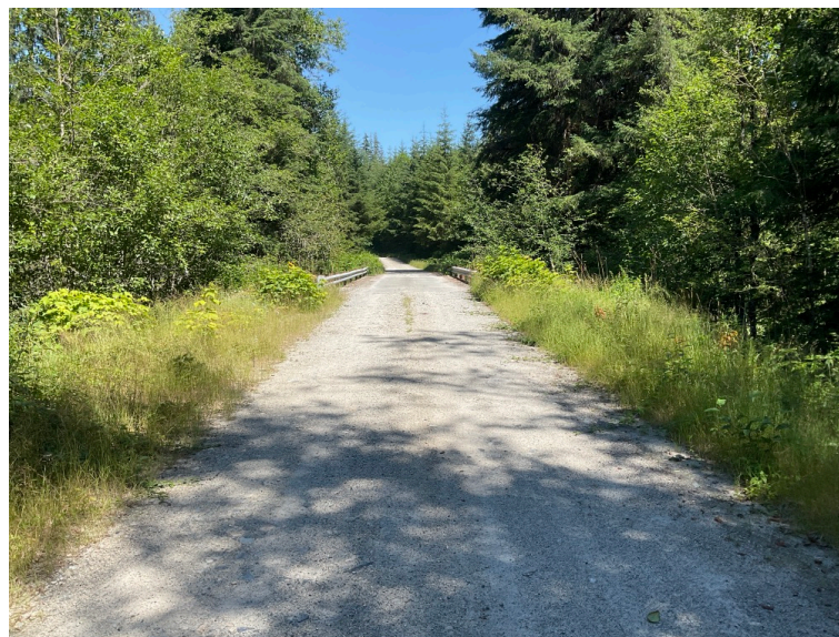
Approach from Right Bank when facing downstream
