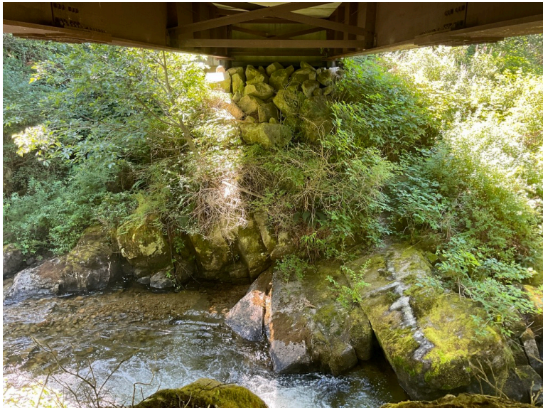
Right Bank Abutment when facing downstream
