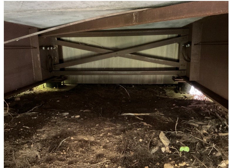
Left Bank Abutment when facing downstream
